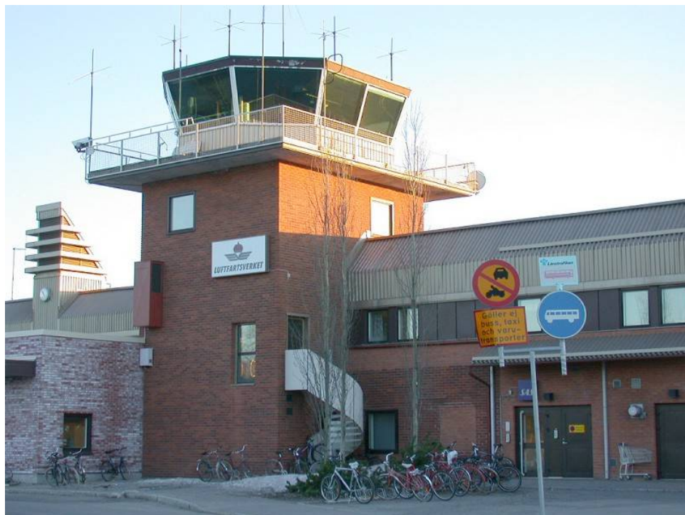
The tower at Umeå airport seen from landside
