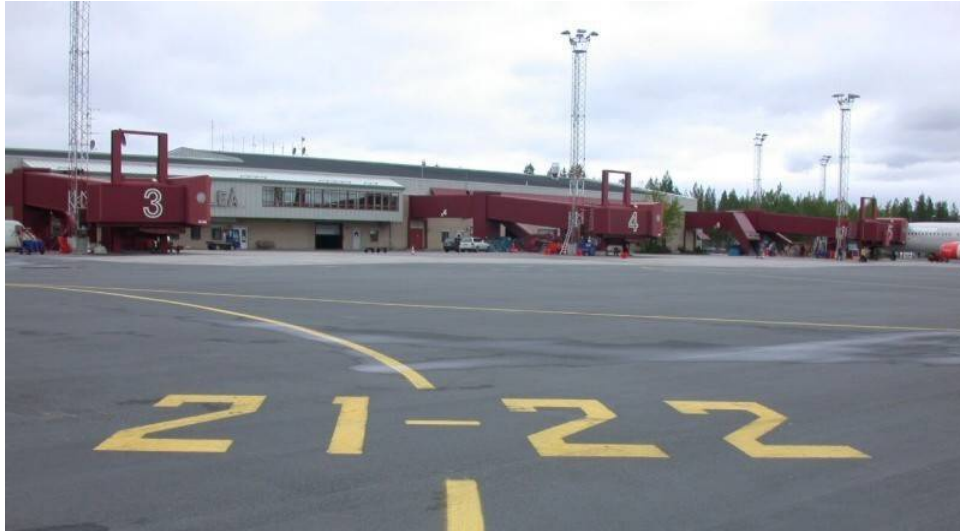
Terminal building at Luleå-Kallax airport seen from Apron 9.
